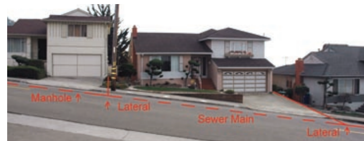
In this photo, the gray house is at risk. The pink house may be at risk if it has a floor drain in the garage. Most likely, the house on the left is not at risk.
