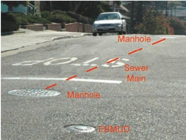
Connect it to the next nearest manhole so that the dotted line passes in front of your house. The main is located under the street at that dotted line.
